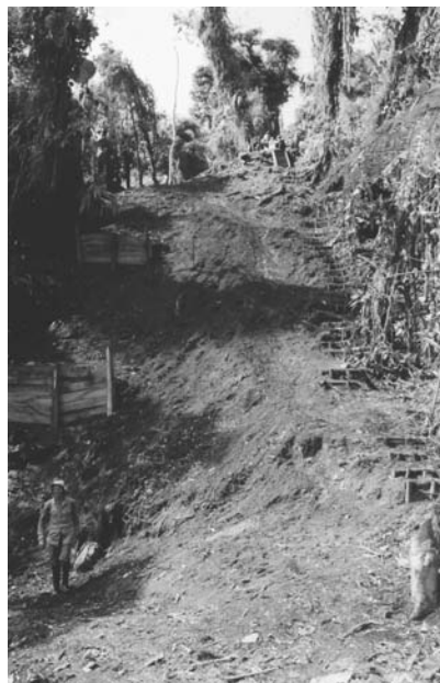
FIGURE 16: The right of way of the underground OCP pipeline varies in width from less than 7 meters in ecologically sensitive zones, such as the Andes Mountain slope in the photo, to 30 meters (Enrix, 2001). OCP passes near six active volcanoes and through seven national parks and protected areas, including a World Bank Global Environment Facility project, managed by Fundación Maquipucuan, and affects potentially an estimated 450,000 people living along its route (Enrix, 2001).
