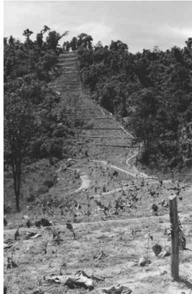
FIGURE 17: Once the OCP pipeline was buried, revegetation efforts with native and nonnative plant species were conducted by Fundación Jatun Sacha. The right of way was not reforested so as not to stress the underground pipeline.
